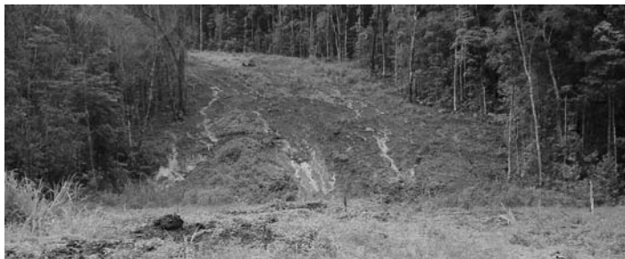
Cleared road with erosion scars, Speewah
